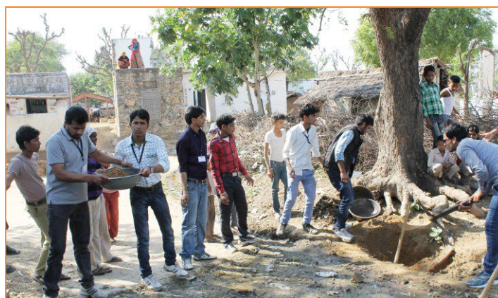
Soak pit construction in village under sanitation drive
