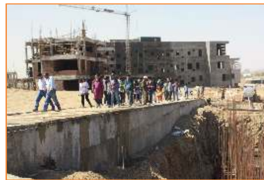
Field visit to Shree Cement Factory, Pali
